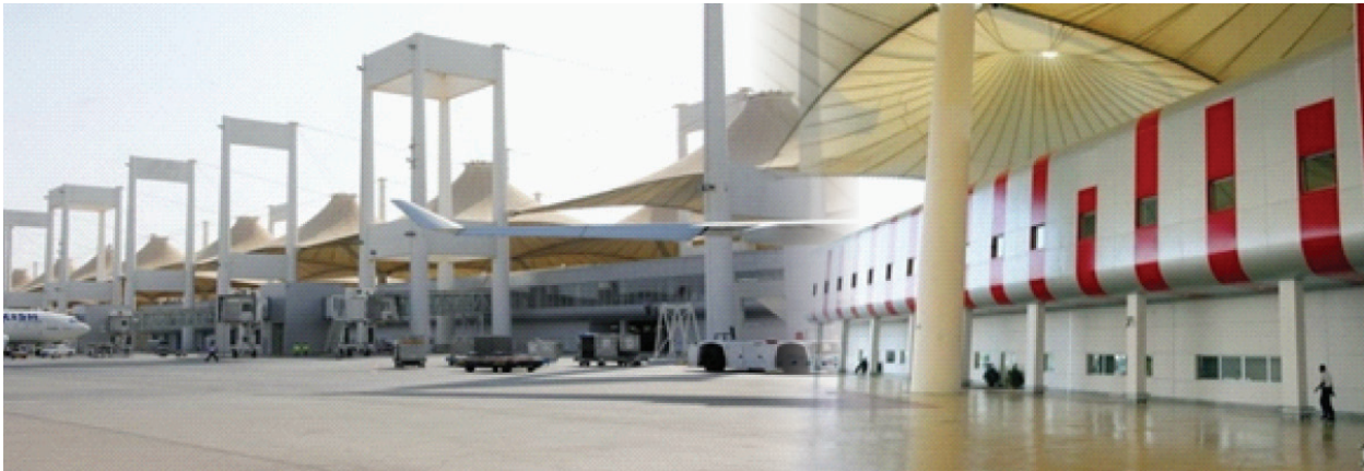
Hajj Terminal completed during 1430H (2009) - with part financing from IDB, Jeddah, Saudi Arabia
