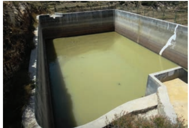
Overview of the rainwater harvesting reservoir for irrigation (Low water level during dry season)
