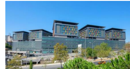
IsDB-funded Okmeydani Training & Research Hospital
