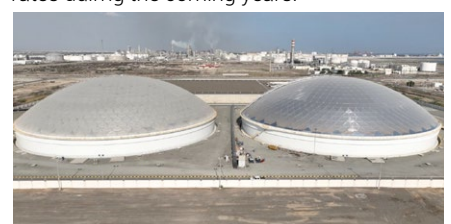
Water reservoirs at Sohar Desalination Plant
