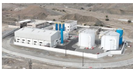
Pumping Stations on the pipeline route
