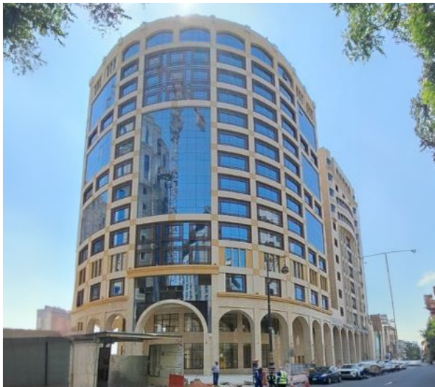
19: Albayan Foundation's Vision Realized: Construction of a Hotel in Al Madinah
