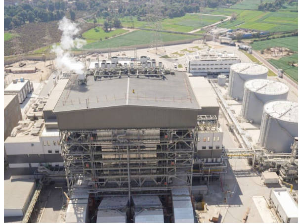
6: Boiler Overview - Assiut (El-Walidia) Thermal Power Plant Project
