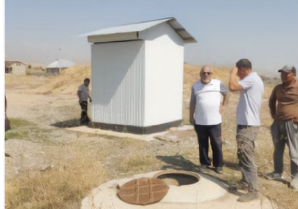
8: Water Wellfield at Besh-Moinok Subproject, Suzak District - Rural Water Supply and Sanitation Improvement Project
