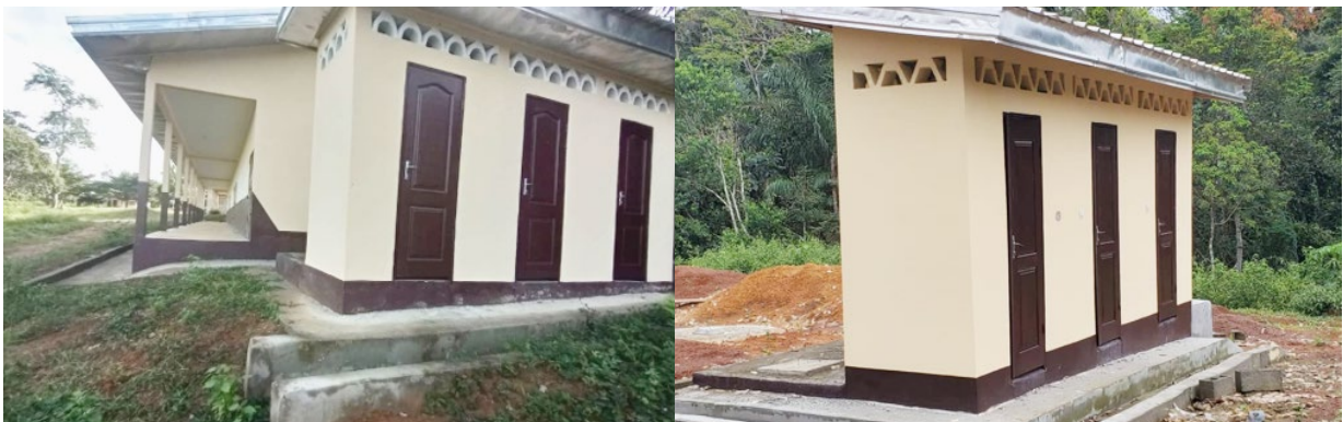
4: One block of Three (3) Latrines – Olama - Kribi Road Project - Construction of Olama-Bingambo SectionII)
